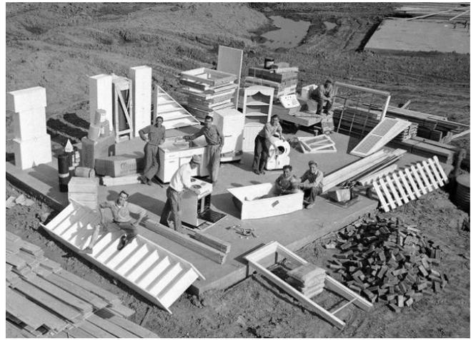
**Figure 4: A specialized crew poses for a photo while installing cabinets and appliances for a Cape Cod house in Levittown, NY. Many parts, such as cabinets, staircases, and fences were pre-fabricated and assembled on site. Source: Getty Images**
